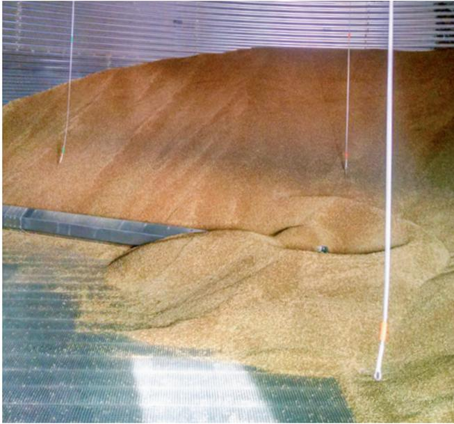
*These sensor cables inside a wheat bin at Arrow K Farms assess temperature and moisture. The information is reported and recorded electronically through a system developed by IntelliFarms. Then, the Kessels can open an app on a mobile phone or personal computer, and learn the findings — and even change the fan settings.*
